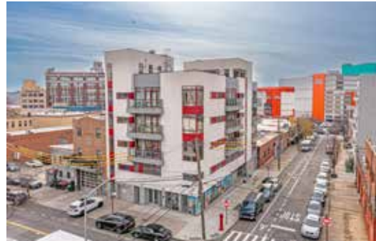
32-04 34th Street, Queens $11,244,000
